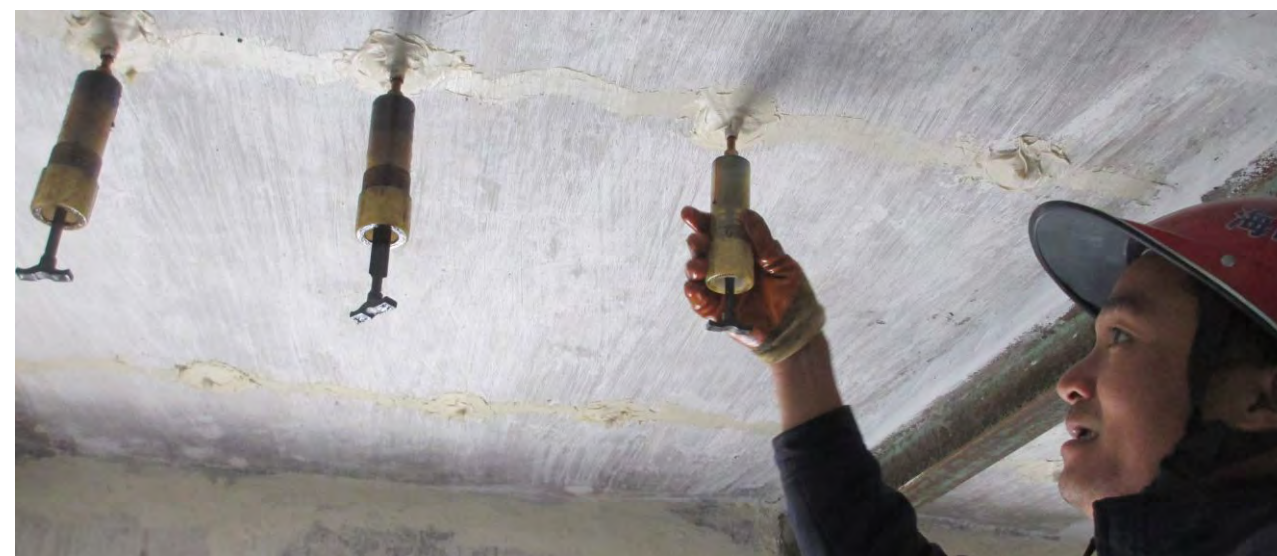
积庆楼修补裂缝
